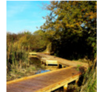
Timber deck & boardwalks to allow for access to the SuDS features.
